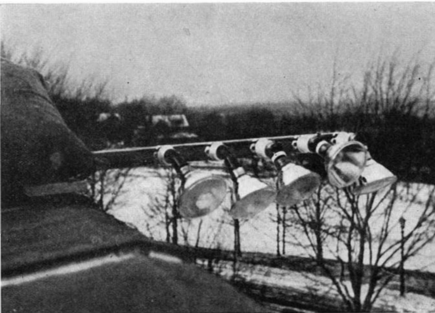
Another way of using projector lamps, employing adjustable sockets
