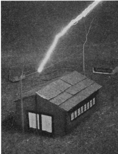
Model lightning shield stands test
