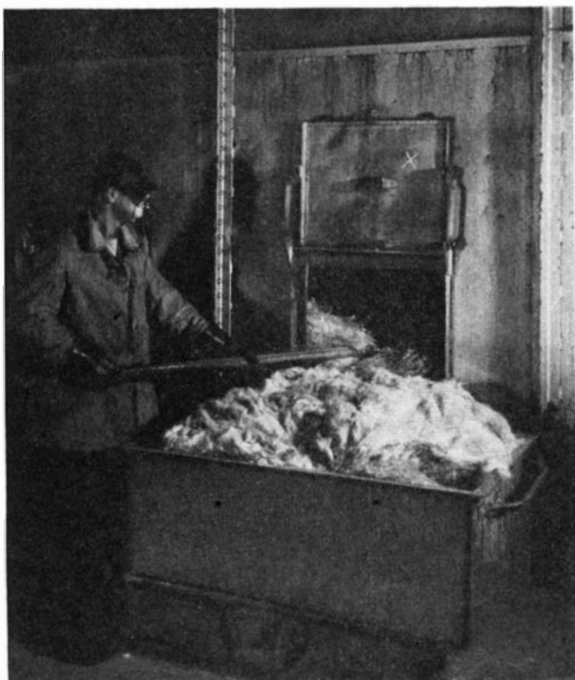
Removing crude phthalic anhydride from a condensing bin. This chemical, made by oxidation of naphthalene, which in turn is derived from coal tar, is an important intermediate in manufacture of smokeless powder, dyes, and certain resins
