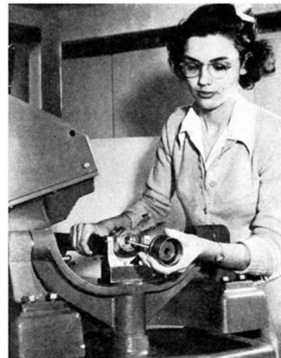
Inserting the Garand bore plug
