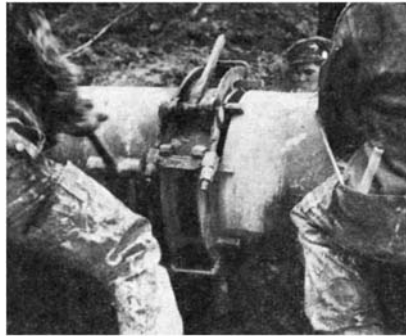
Along the "Big Inch." Upper left: Men of the tie-in crew stand on pipe to bring the ends into line. Above: Lining up and clamping a section of pipe to the end of the line. Below: Putting the last pass of a roll weld on one section of the "Big Inch"
