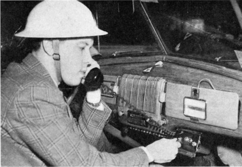
The radio in this Auxiliary Police car has been converted into a shortwave WERS set, permitting maintenance of constant two-way contact with the control center
