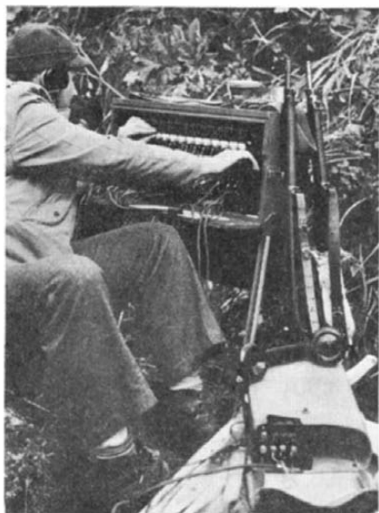
First ashore—a field switchboard
