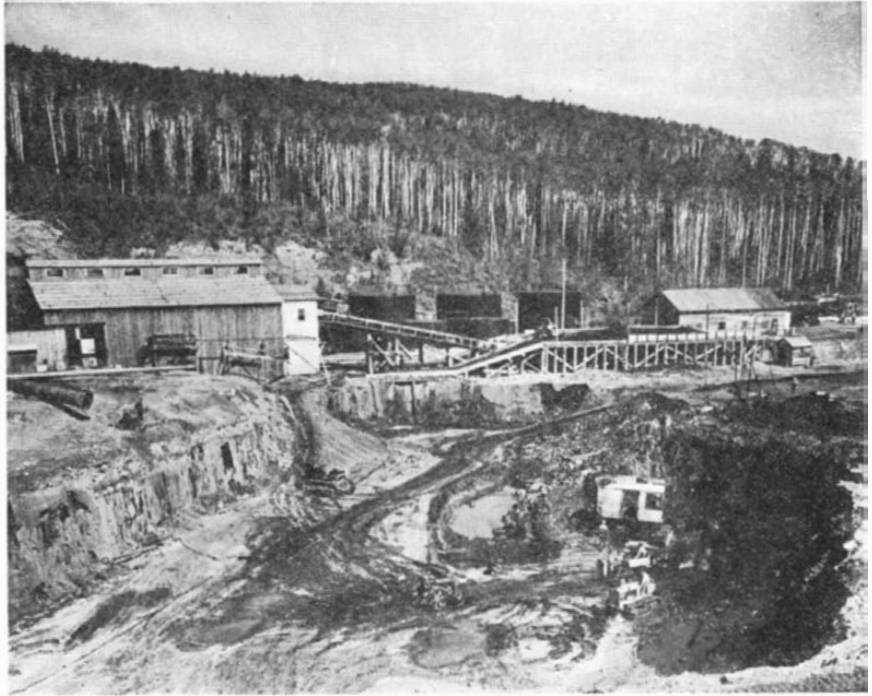
A general view of the open-pit mining area at the McMurray, Alberta, pilot plant, where oil-sand deposits are found at a depth of 15 feet below the surface
