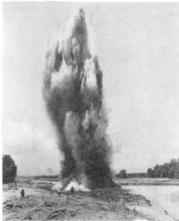
Dynamite blasts a new channel for a stream
