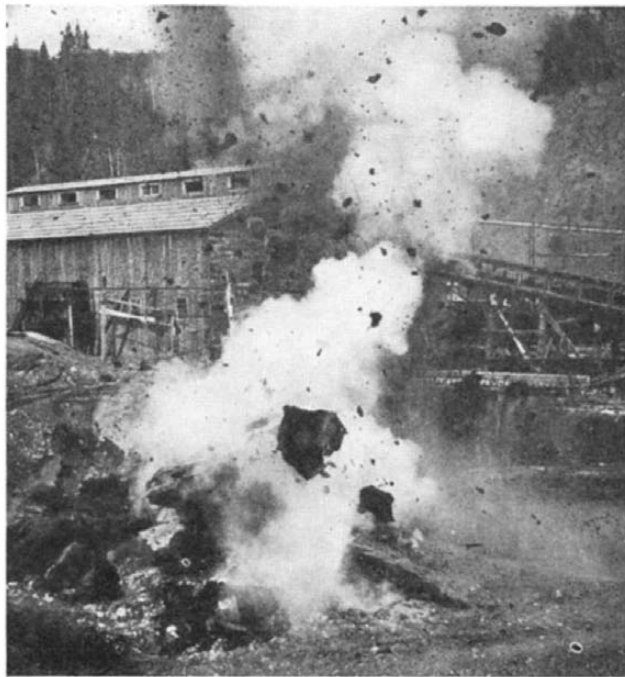
Blasting out sub-surface oil deposits
