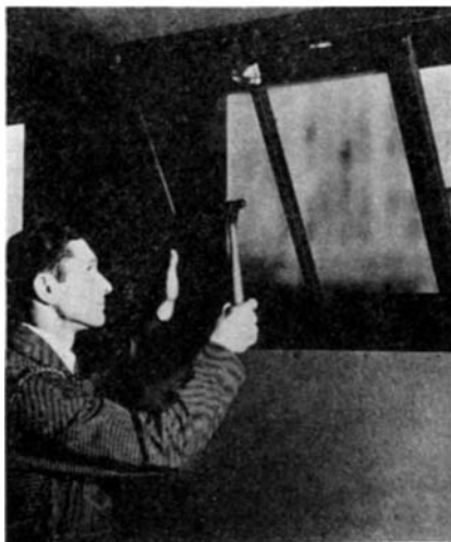
Glazing material which may be installed with a hammer is composed of a shatter-proof plastic and wire. It is also used where possibility of explosion makes glass dangerous
