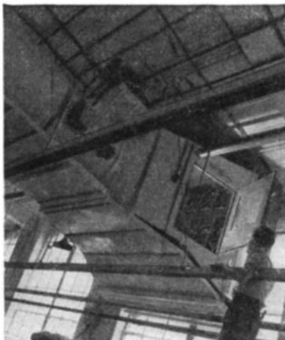
Cleaning duct in a textile mill
