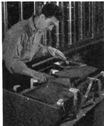
Charging wires and discharge plates of an electrostatic-type air cleaner
