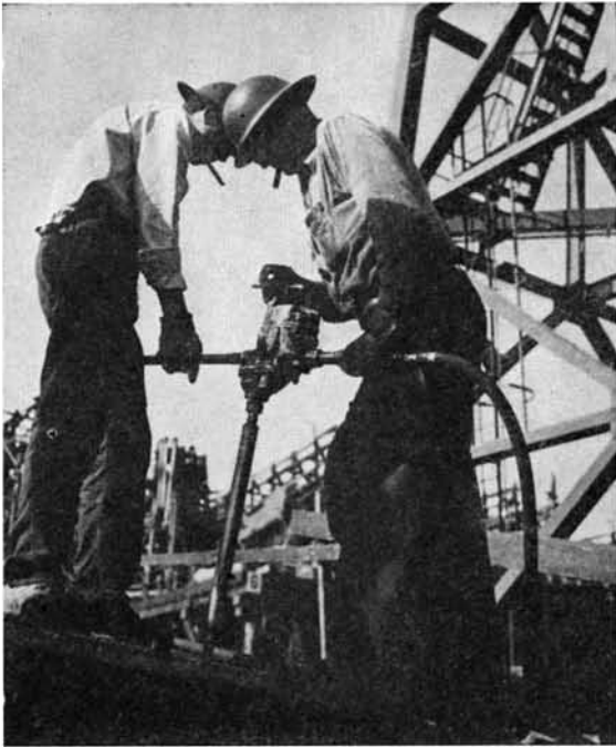
Air-driven reamers truing holes in ship construction
