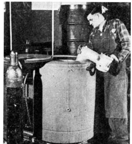
Cold-shrinking the male part of an airplane landing strut assembly
