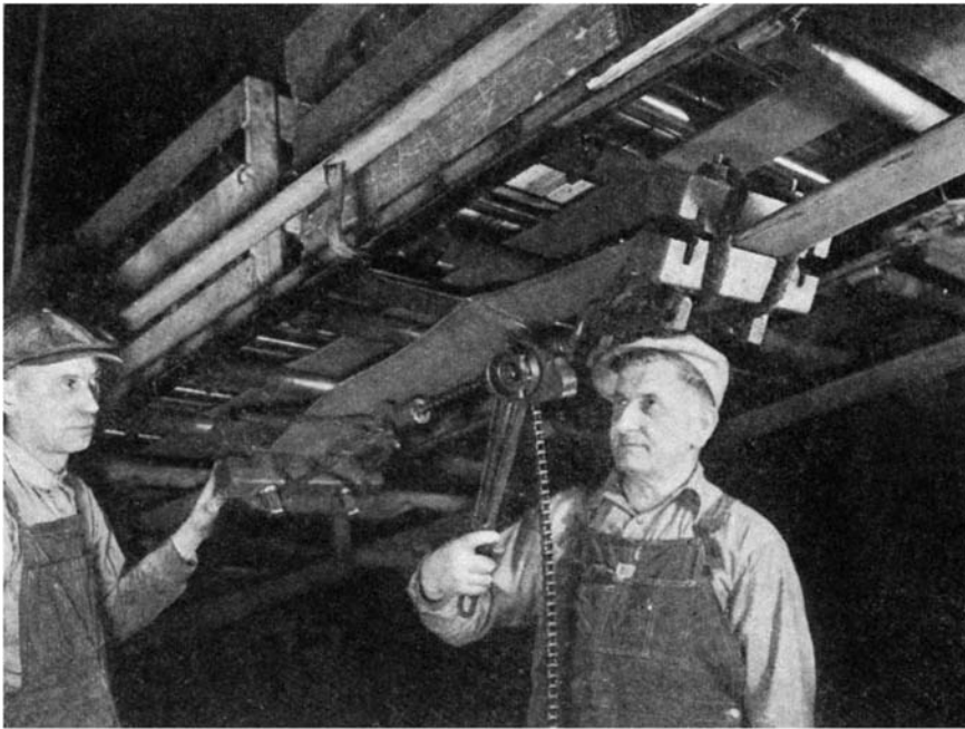
Hooking up a live roller conveyor drive belt
