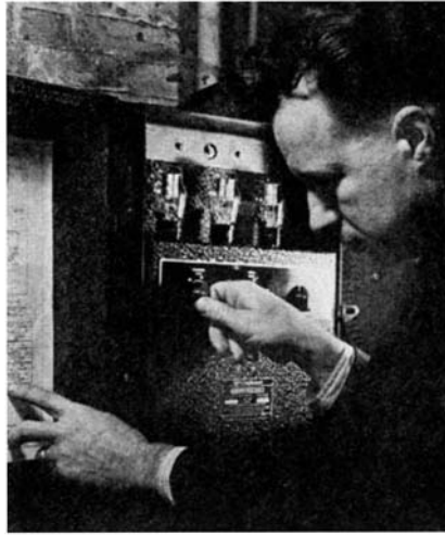
Electron tubes in this set-up automatically time the duration of the current used for resistance welding
