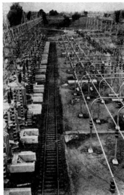
First recorded installation of welded wrought-iron electrical buses
