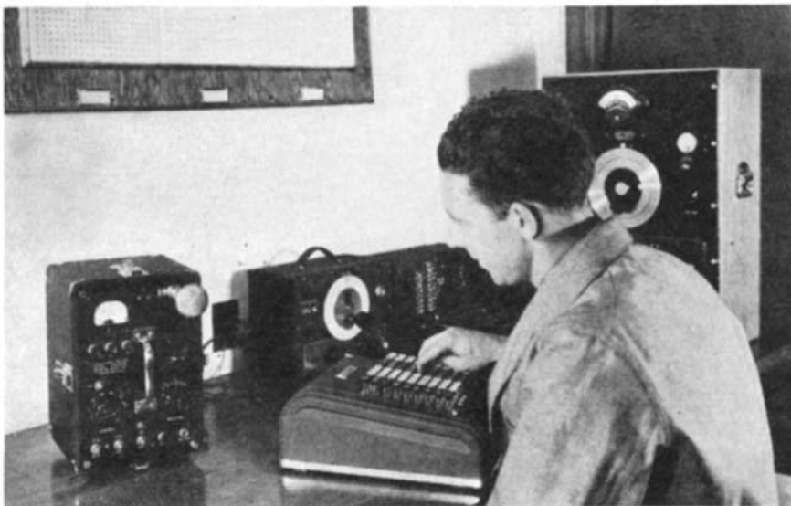
Checking noise on a new comptometer model, made quieter through research
