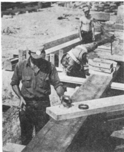
Formerly the Achilles' heel of timber construction, joints are now strengthened with ring connectors. Those shown are of the split type fitting grooves cut into the timber
