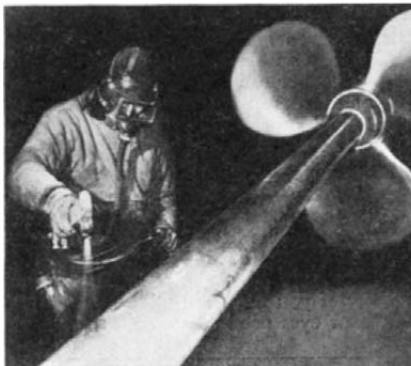
Flame-spraying Thiokol onto a propeller shaft to prevent electrolysis
