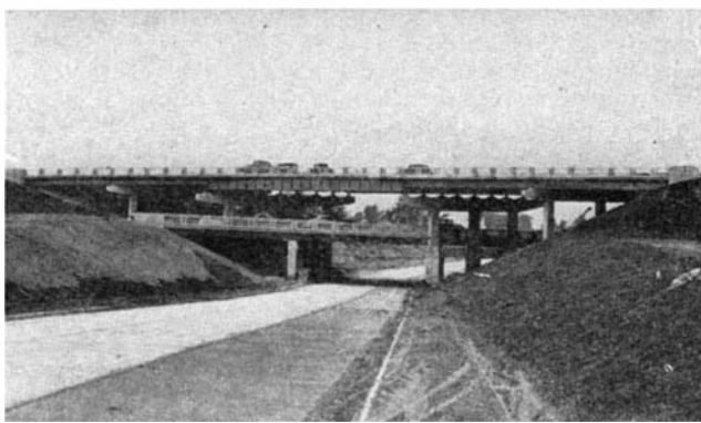
A three-level crossing at the Ford Willow Run plant on the Detroit Industrial Expressway. This highway was designed as the initial part of a future limited-access road
