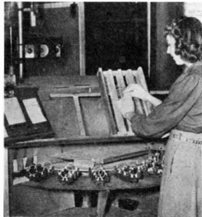
One of the rotary-type heating and chilling units mentioned in the text. Note radial rotating arms below. Each arm carries three lenses through an electric furnace
