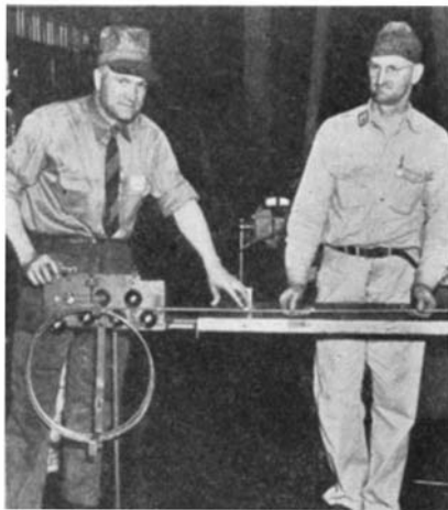
Worker-devised tubing straightener
