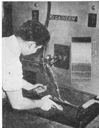
Production-line heat-treating set-up and, inset photomicrograph of hardened surface of a bearing pin
