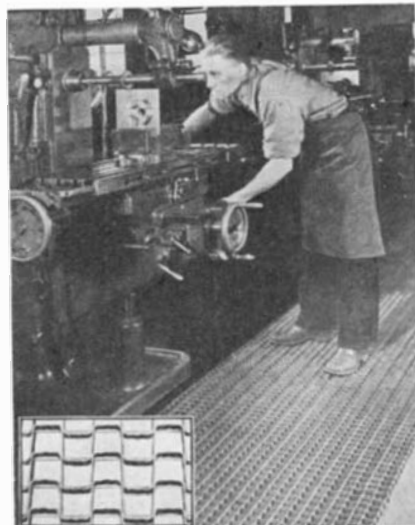
Steel mat (inset) promotes safety
