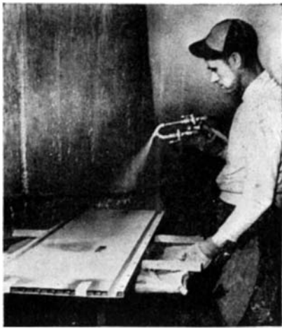
Skid-proofing a catwalk section
