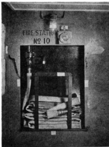
Phosphorescent marking tape identifies a fire-fighting station
