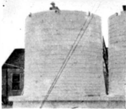
Chemical tanks can be quickly assembled from precast concrete slabs
