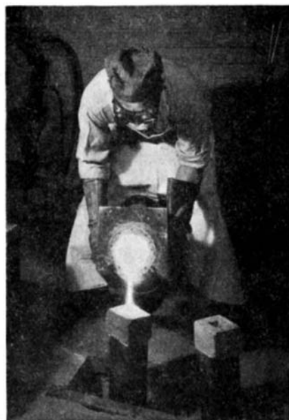
Courtesy Rustless Iron and Steel Corporation Pouring a test ingot
