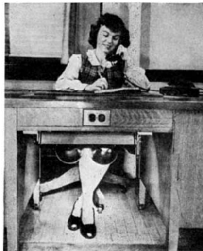
Infra-red lamps, placed under desk, keep the office worker comfortable
