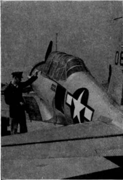
The first BT-15 airplane to employ "sandwich" type of glass-plastics construction for such structural parts as the rear section of the fuselage, tail cone, and side panels
