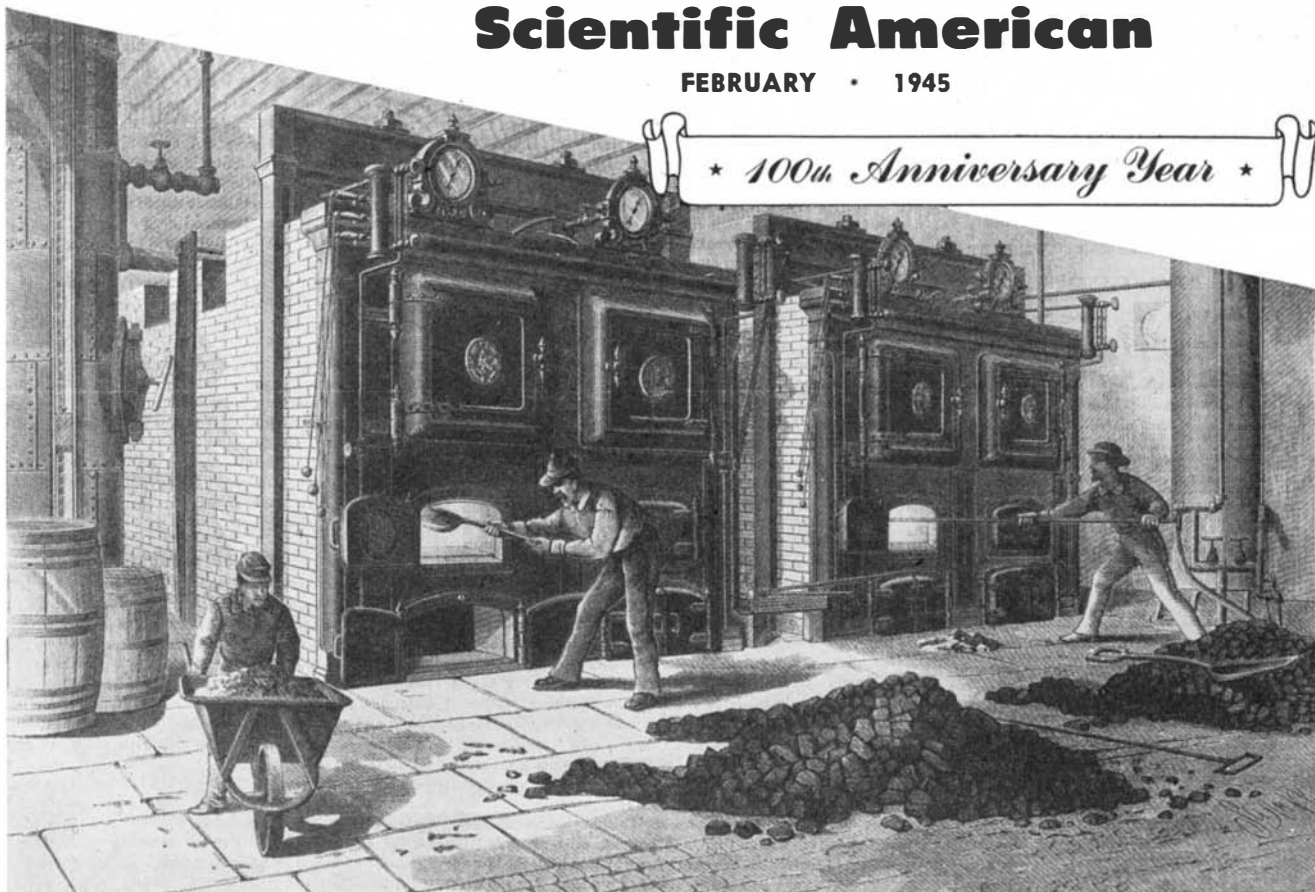
An installation, in 1880, of Babcock and Wilcox boilers in a Standard Oil refinery
