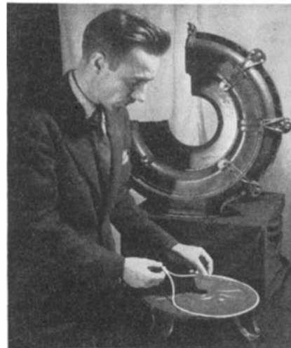
How gaskets of the new silicone rubber, developed by General Electric research laboratory, are applied to the casing of a turbosupercharger
