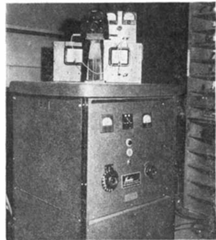
X-ray equipment for lowering frequency of quartz oscillator plates
