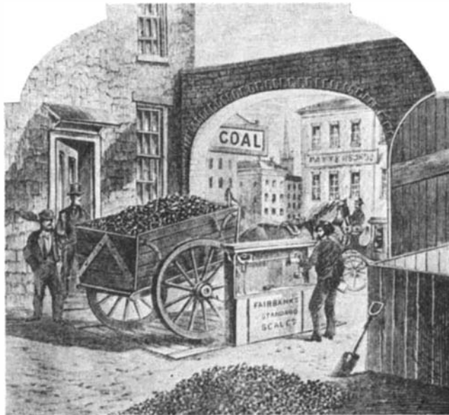
An early Fairbanks platform scale. These weighing units made possible the first steps in providing accurate quantitative control of industrial production
