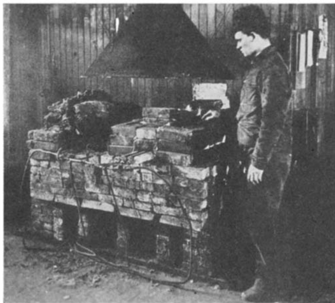
In this crude electric furnace, Dr. Edward Goodrich Acheson conducted experiments in the 1890's in the production of the now widely used Carborundum
