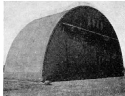
Vynylite-impregnated canvas over a steel frame makes a portable hangar
