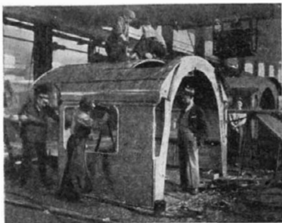
Left: Cabs of aluminum alloy being fabricated for use on high-speed steam locomotives Courtesy Aluminum Company of America
