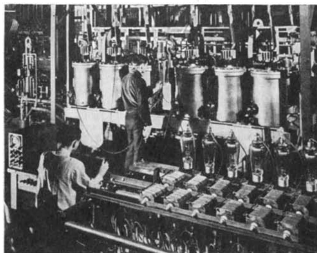
Shop-testing a huge ignitron rectifier assembly that is now being used in the electrolytic production of aluminum
