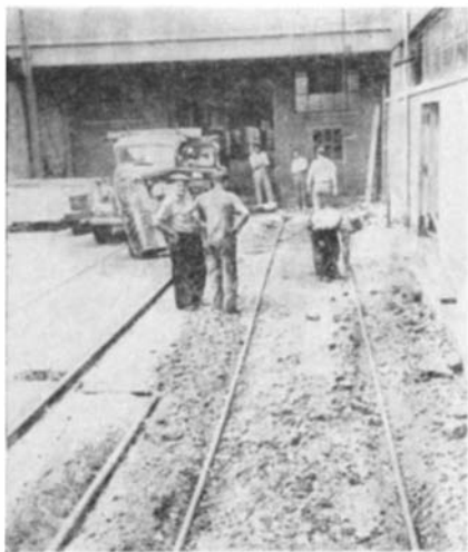
Installing wrought-iron pipe coils for melting the snow by radiant heat
