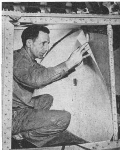
Sheets of impregnated glass cloth are used to line fuel-cell cavities
