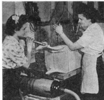
A vacuum cleaner withdraws the air; the heating unit seals the package
