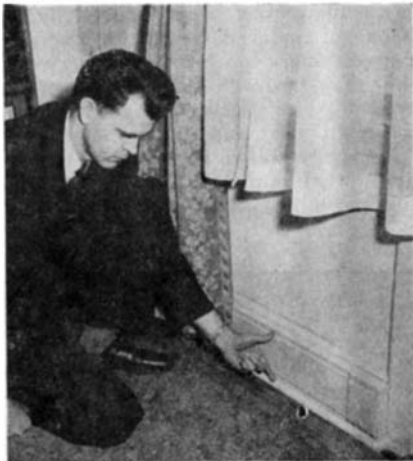
Left: The cast-iron baseboard radiates heat. Above: Cover removed to show pipe connections and vent valve
