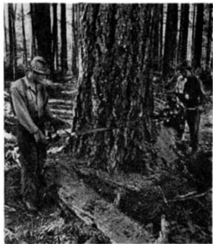
Gasoline powers this chain saw
