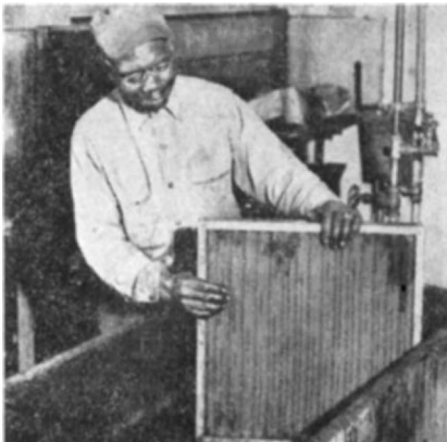
Dipping cleans all air filters
