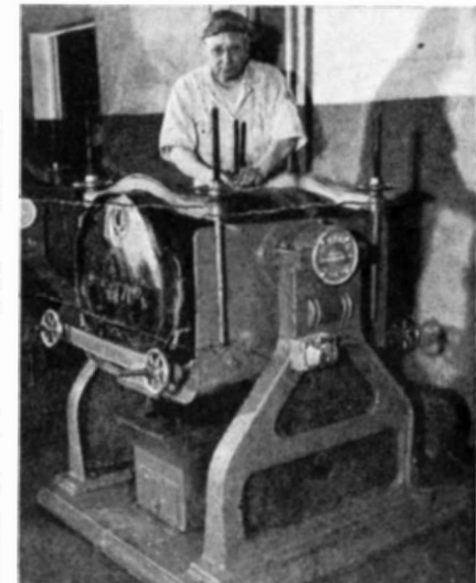
Paint mixer handles 50-gallon drum
