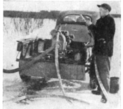
Multi-use pump on a trailer
