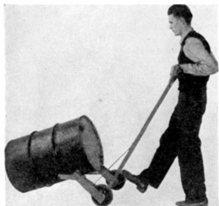
One step in upending a barrel
