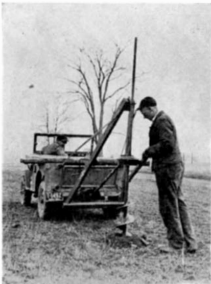
Builds fences in a jiffy. Jeep can carry posts, operate hole-drilling augur, and stretch wire afterwards
