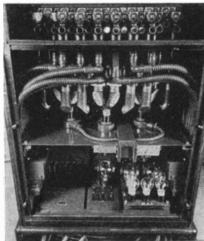
Smoke-detecting cabinet with front panel removed to show the pipes going to various parts of the ship. Large lamp in the center provides the light that actuates the photoelectric cell
