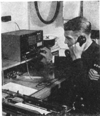
Midget Western Electric radio-telephone set installed on a merchant-marine training ship. Units like this are also widely used on pleasure craft
