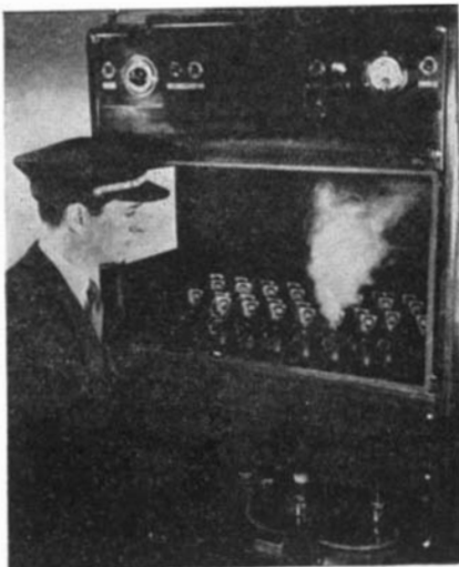
The number on the outlet from which smoke emerges in the Rich-Audio fire detection equipment for ships shows the location of the fire. At the same time, the smoke interrupts a light beam to a photocell and an alarm is sounded. Thus smoke can be detected visually, by smell, and by electronics
