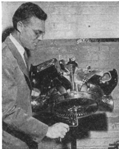
Model of "hat-box" supercharger
