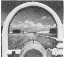
Our Cover: Tank "farms" located near oil refineries are studded with metal storage tanks containing from 55,000 to 140,000 barrels each. In foreground of our cover is a pump and by-pass, the "heart" which controls the flow of oil to and from the tanks. Courtesy Standard Oil Company (New Jersey)
