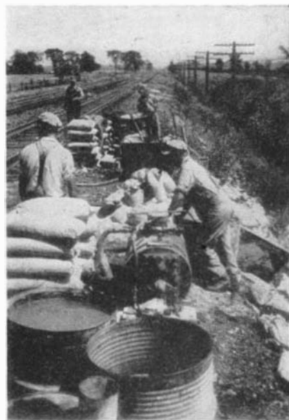
Two crews at work grouting soft spots in track of New York Central System
