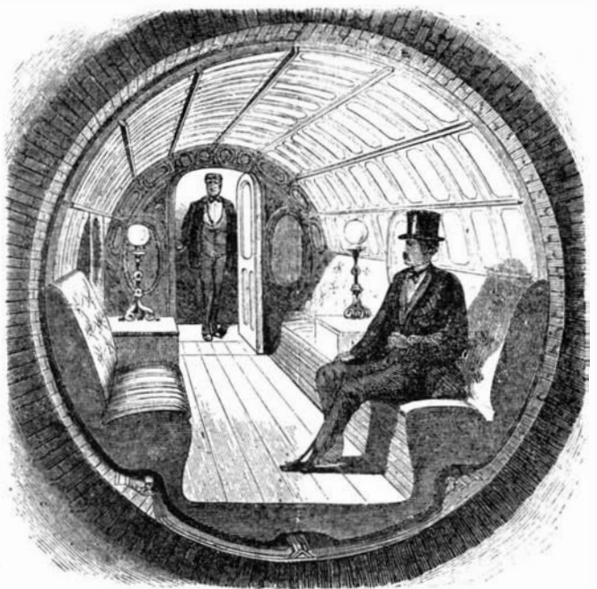
The doors of the Beach Pneumatic Transit Company were opened to the public on February 26, 1870. At left is a view of the tunnel and at right a section of one of the cars that were driven by air from "a gigantic blowing engine"
