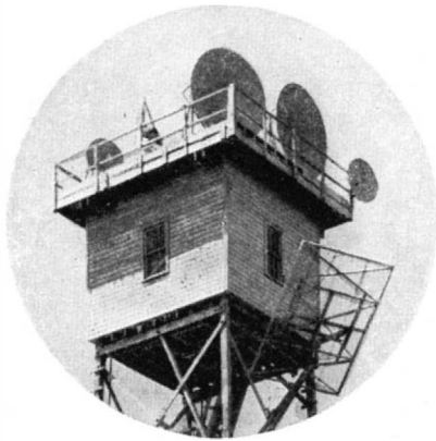
An antenna installation for the pulse time modulation multiplex radio relay system developed by the Federal Telephone and Radio Corporation as a new method of handling microwaves
