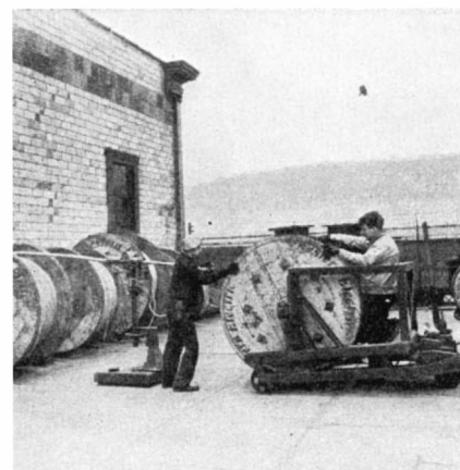
A special purpose lift truck applied to handling large reels of cables
