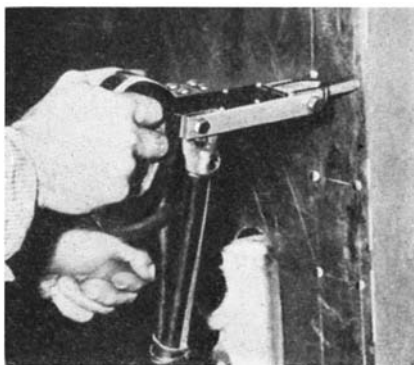
Setting the new explosive rivet
