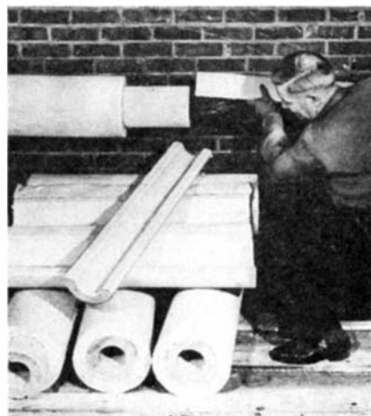
Telescopic installation of dual-layers
