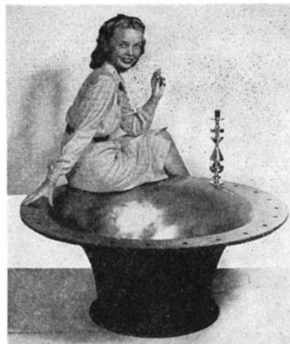
Precision contours for supercharger housing or delicately shaped candlesticks are accurately duplicated from master pattern by "electronic finger"
