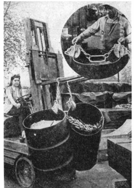
Chain and grips will lift four-ton load
