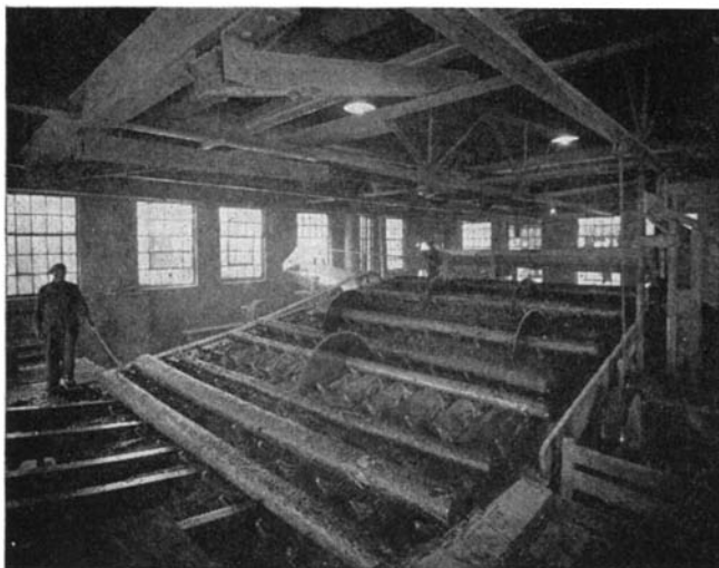
Five-saw slasher (left) and pulp wood grinders (right) are initial steps in wood processing
