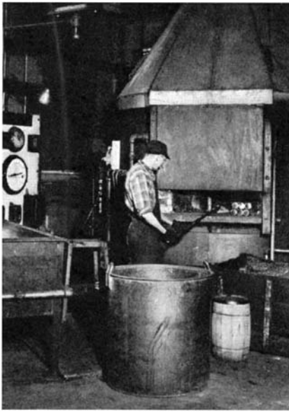
Controlled atmosphere furnaces demand precision controls. Note panel
