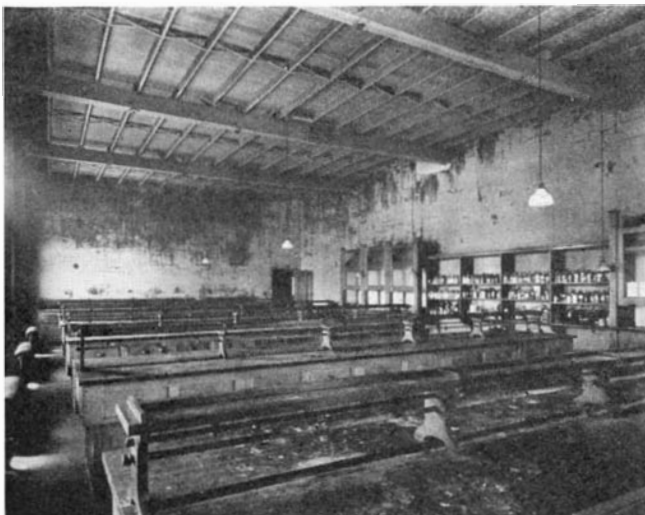
Unpleasant working conditions—laboratory before painting
