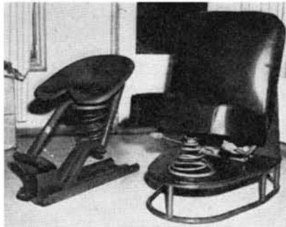
Spring adjusts for driver's weight
