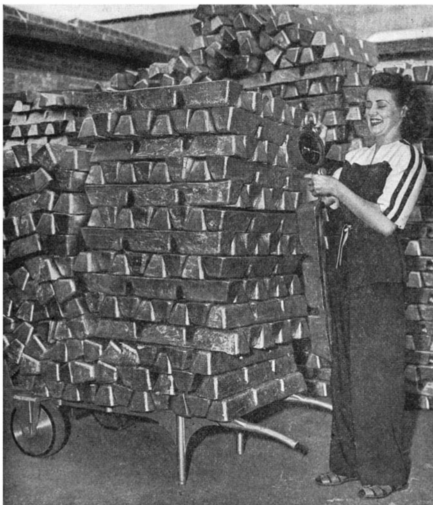
No heavier than one of the 175 aluminum ingots stacked on its chassis, the Northrop Gaines aluminum hand truck, which easily bears the load, weighs only 30 pounds
