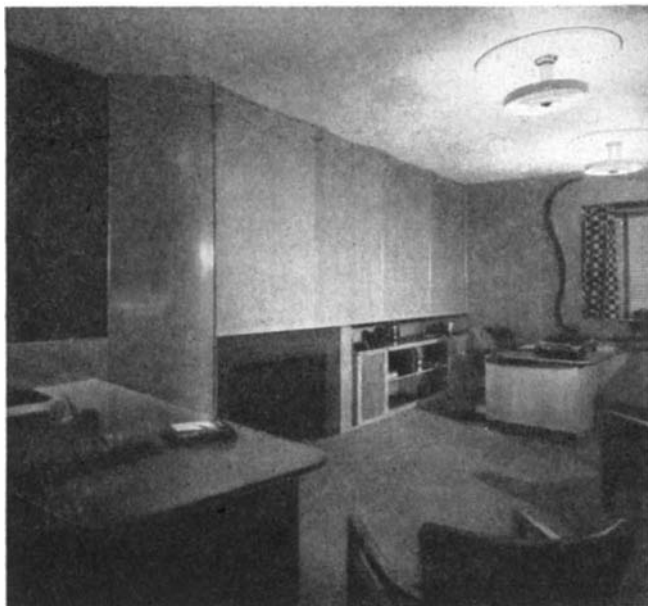
The flexibility of standard quarter-inch plywood is demonstrated by its use in the four concave panels. Eighth-inch stock was required to construct the sharply curving surface
