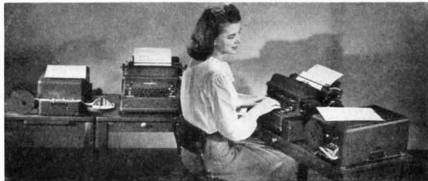
Controlled by the electric typewriter, the automatic perforator at extreme right records on a narrow paper tape the body of a letter to be reproduced
