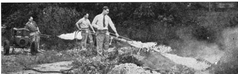
Above: Close-up of the power burner with two torches in brackets on the side. Left: The burner in use, operating three four-gallon-per-hour torches. Note length of flames and large working radius possible
