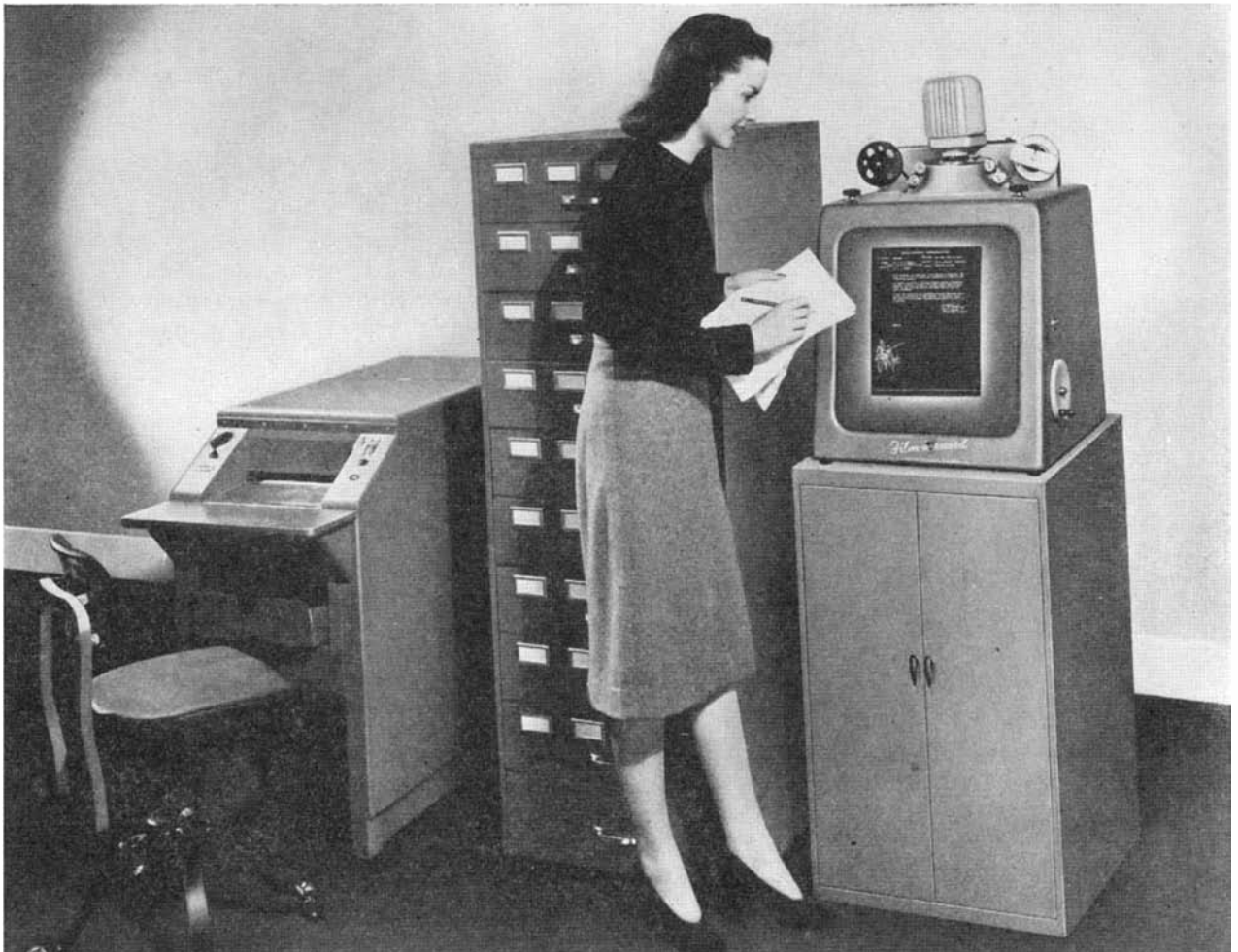
A complete office set-up for microfilming—film recorder, file equivalent to 160 four-drawer cabinets, and reader
