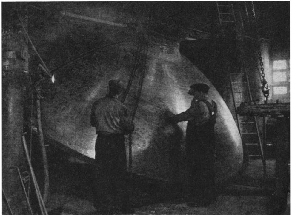
At left and right are views taken in the George Keller Copper Works, Brooklyn, New York, one of the largest fabricators of brewery and other processing equipment. Here copper is shaped to required forms in huge sheets and tubes, much of the work being of such a specialized nature that it is done by hand
