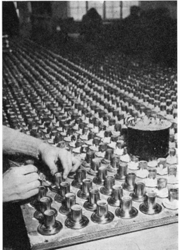
Parts set up for mass fluxing and silver brazing
