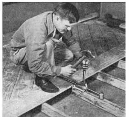
Floor-laying tool in use
