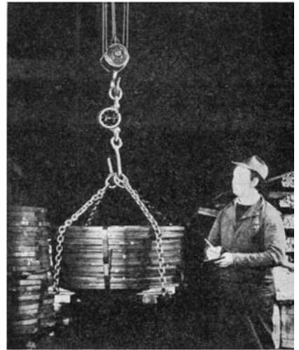
Scale is between load and hoist hook
