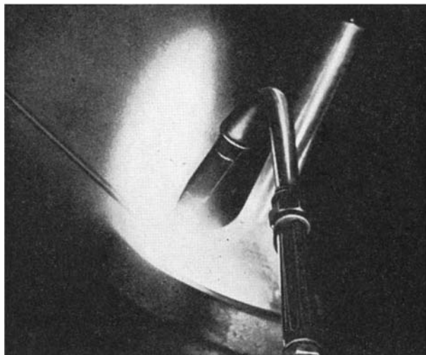
Hard-facing with an oxyacetylene torch gives a good bond with a minimum of weld penetration
