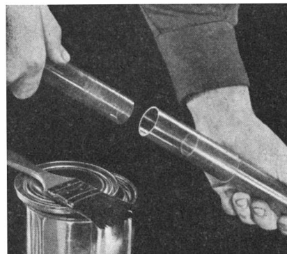
Joining two lengths of plastics gas pipe
