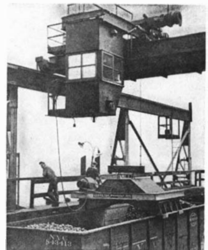
The shakeout in position astraddle a hopper car which is to be unloaded
