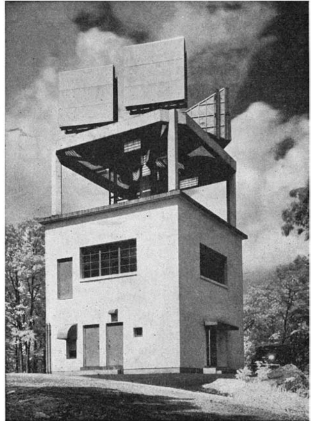
One of the stations in the microwave relay links between New York and Boston. Directional antennas are mounted on roof
