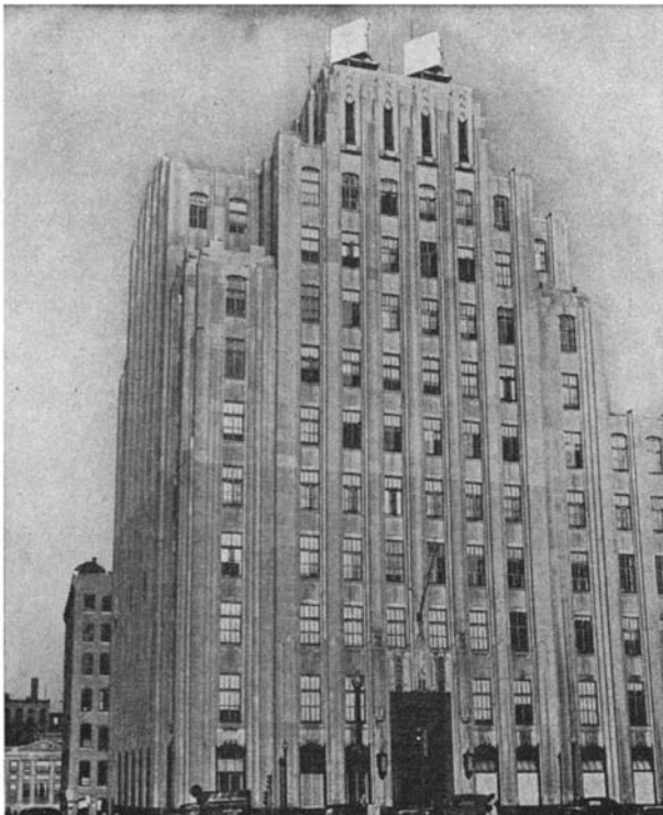
The Bowdoin Square Building, which is the Boston terminal of the Bell System's New York to Boston microwave relay route. The antennas can be seen at the top of the building
