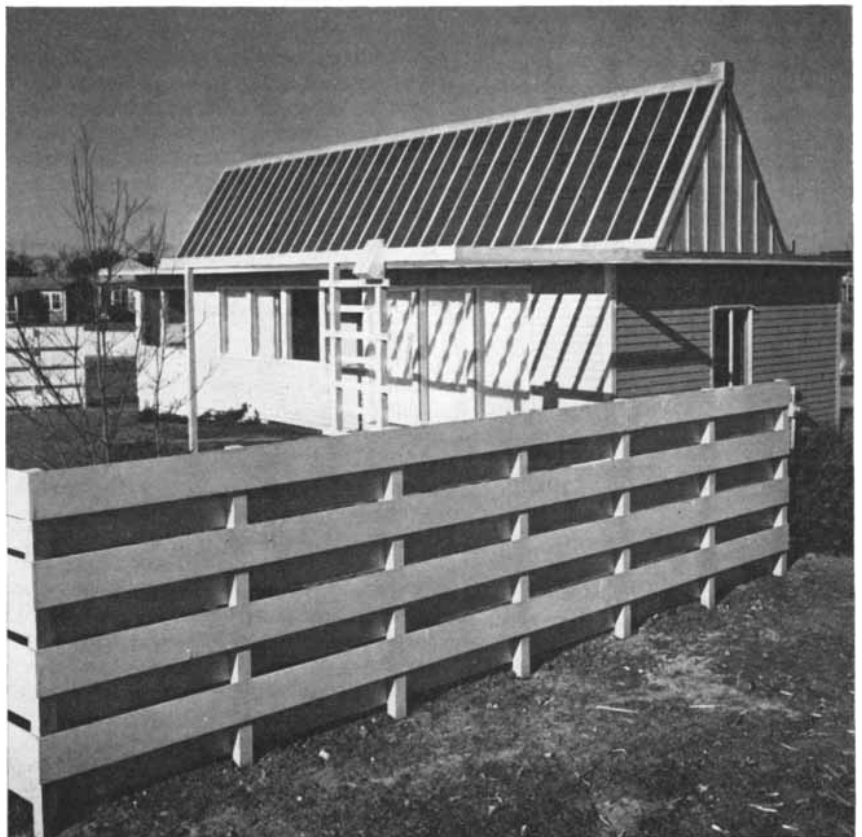
M.I.T. HOUSE in Cambridge has heat collectors on the roof. The heat of this house is stored in water; of the Dover house, in Glauber's salt.
