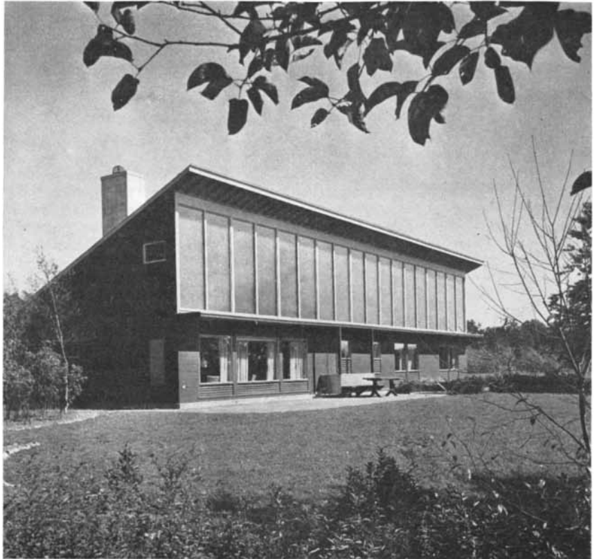
DOVER HOUSE in Cambridge, Mass., is heated by solar energy. What appear to be large windows in the second story are glass heat-collectors.
