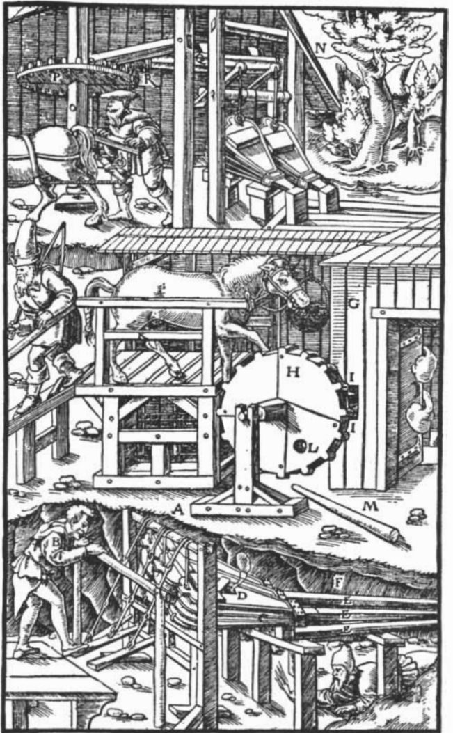
VENTILATION of mines was a serious problem. Sometimes it was solved by a magnificent arrangement of bellows. These were operated by horse- or manpower.
