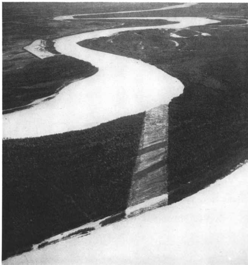
JACKSON CUTOFF eliminates a bend in the river. When this photograph was made in 1939, the trees had been cleared from the zone of the cutoff.
