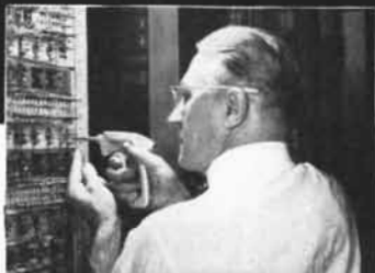
Bell Telephone Company craftsman wraps a wire to complete a connection. Wire is inserted into the nozzle and a rotating spindle whips it around terminals.
