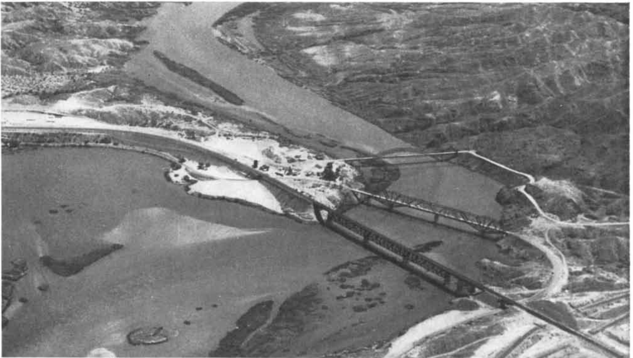
PIPELINE BRIDGE of the El Paso Natural Gas Company, the uppermost of the three bridges shown in this
