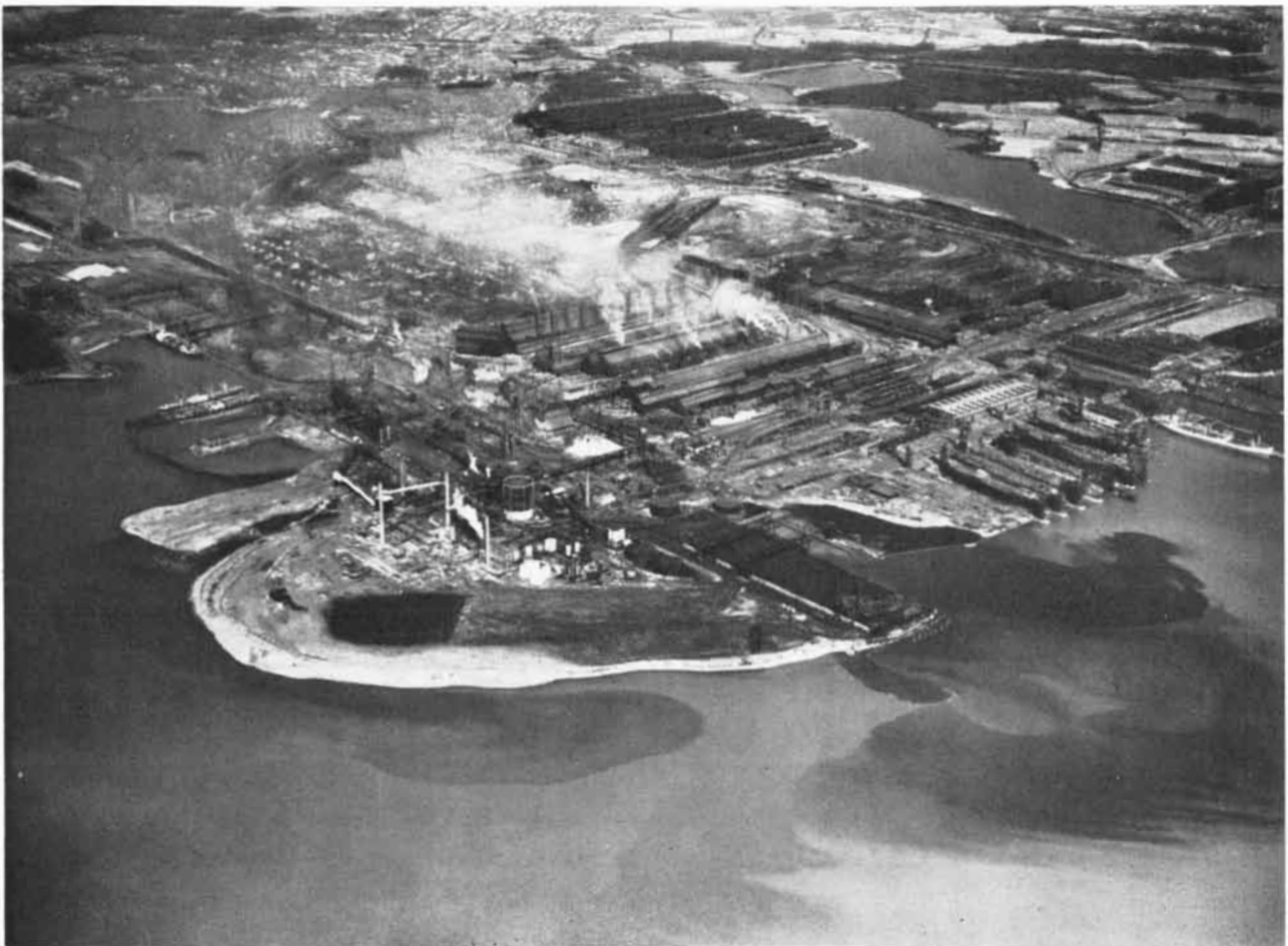
SPARROWS POINT PLANT of Bethlehem Steel is already using iron ore from Venezuela. Its blast furnaces are to the left of the buildings in the center. In the foreground are facilities for storing raw materials.
