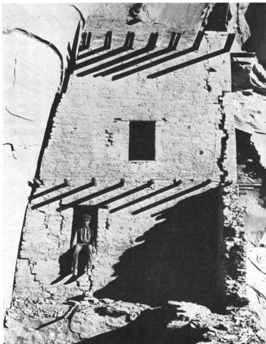
TOWER IN MUMMY CAVE shows how beams are preserved in some Southwestern ruins. The comparison of beam rings has dated ruins back to A.D. 11.
