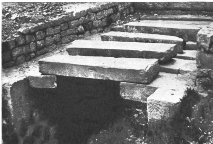
CULVERT in Cusco shows how the Incas built these structures. Although the Incas did not possess the wheel, their highways were paved with fitted stones.
