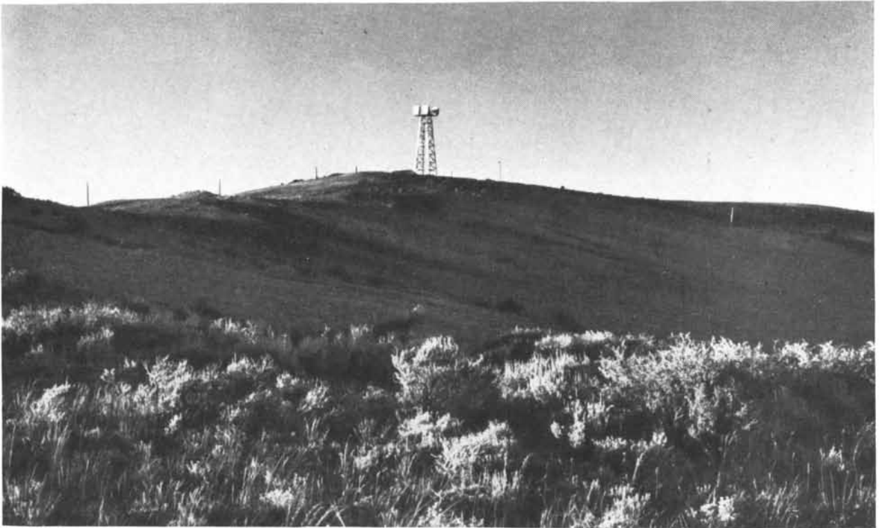
Radio-relay station at Evanston, Wyoming
