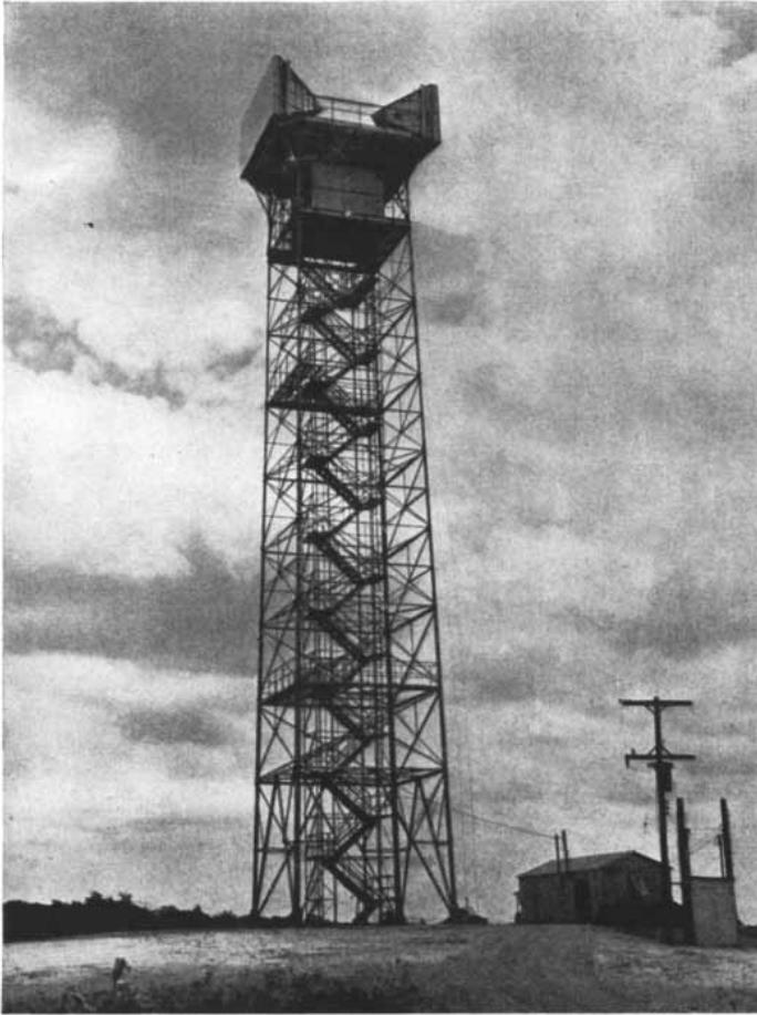
TALL TOWERS support the transmitting and receiving antennas of the American Telephone and Telegraph Com-
