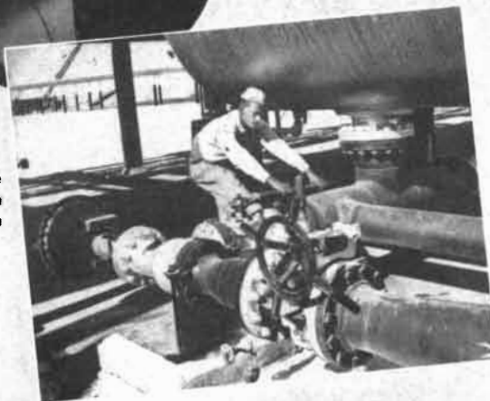
Hammel-Dahl 8" Angle Valve controlling oil level on Separator installation in Saudi Arabia.
